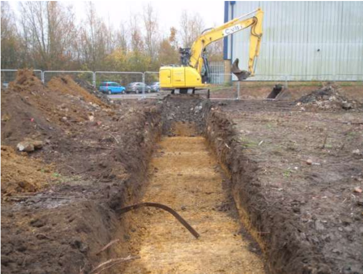
Plate 1. Trench 2 being excavated (looking SSE)
