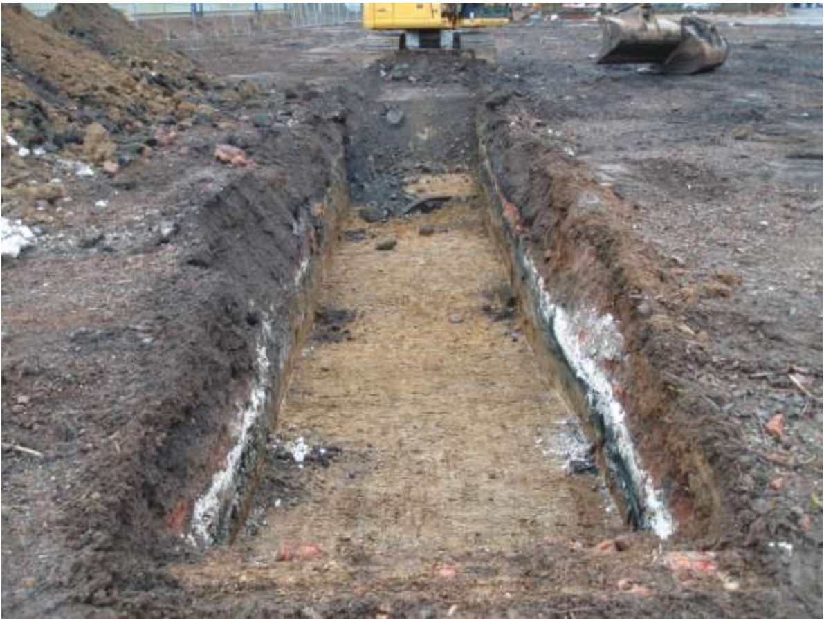
Plate 7. Trench 7 (looking NNW)
